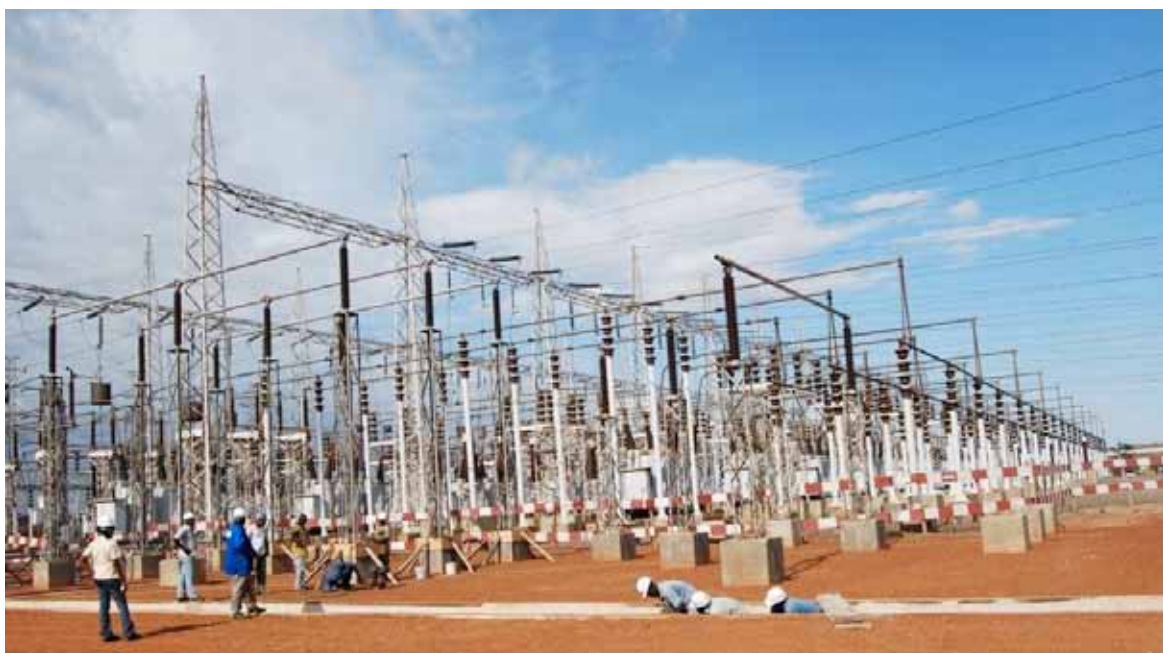
THE VOLTA SUBSTATION EXPANSION PROJECT IN PROGRESS
